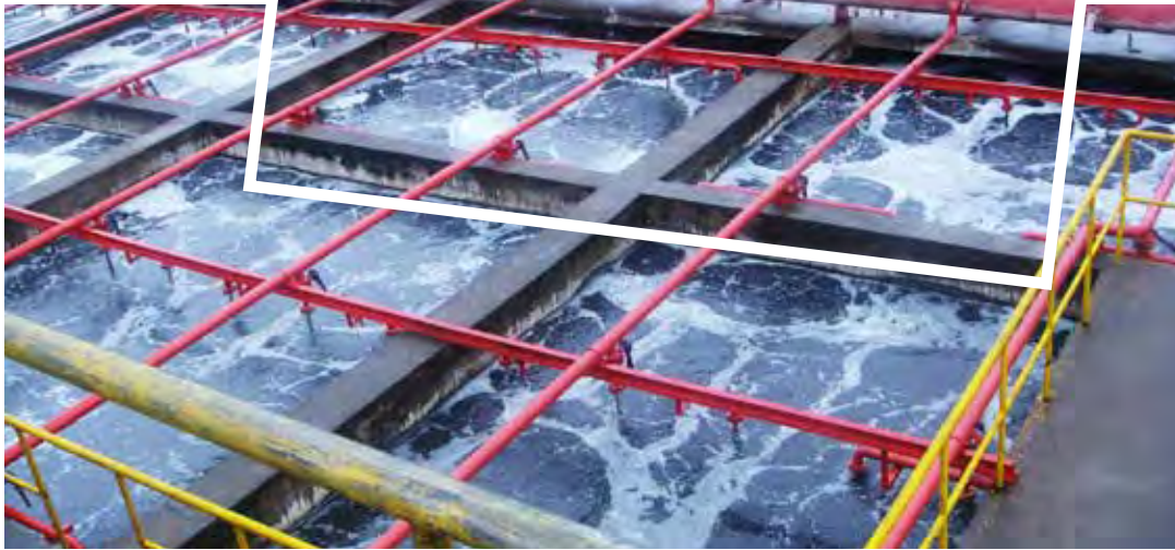
This picture exhibits the aerobic process of a typical waste water treatment plant in a dyeing mill in China that produces fabrics for PUMA products
